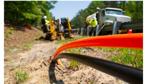
**CLASS-LEADING CYCLE TIMES.** The D40x55 S3 features a carriage speed of 188 ft/min (57.3 m/min) — which is 7% faster than its predecessor, the D36x50 Series II — helping contractors install more linear feet per day.
